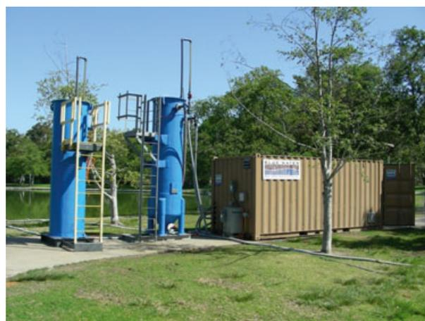
**Fig. 1.** Temporary Blue Pro™ water treatment facility at Mason Lake, April 2008. In a permanent facility, the sand towers can be embedded in the ground, and the trailer can either be camouflaged or decorated as an attraction for public education.
